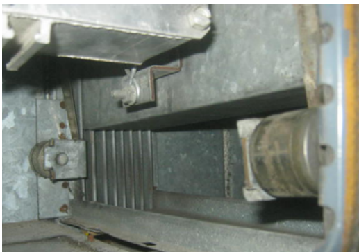
Figure 12.37 Accordion damper
