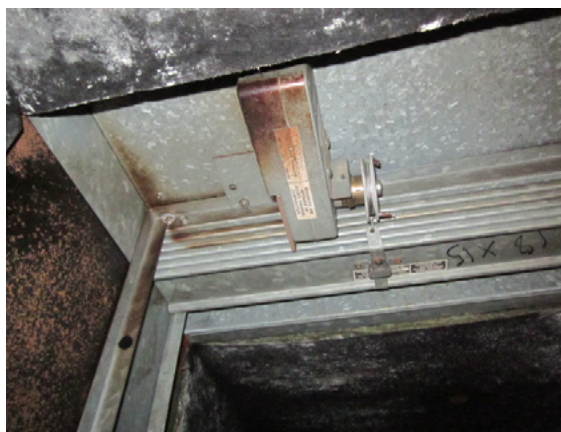
Figure 12.38 Cable connected curtain damper
