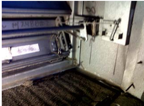
Figure 16.1: Damper blade switch assembly
