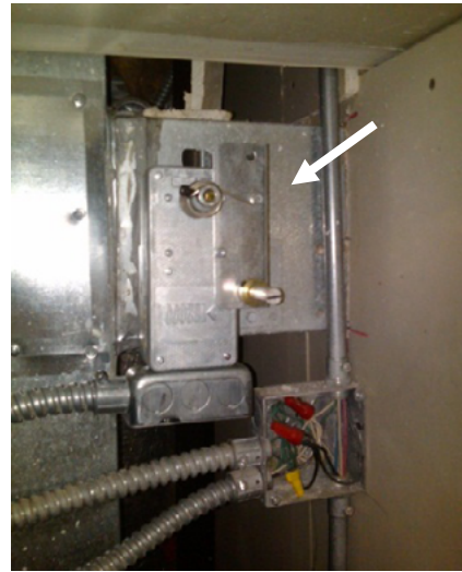
Figure 12.6 Arrow points to the damper shaft.
