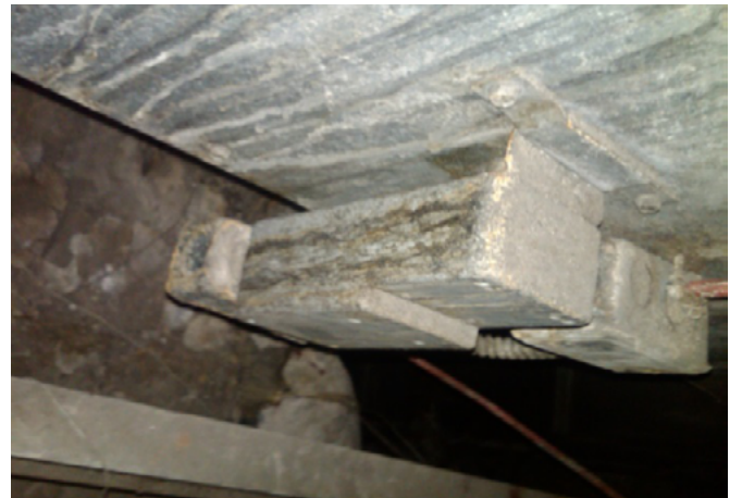
Figure 3.21: External view of motor attached to duct
