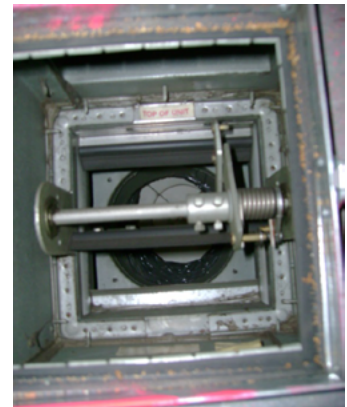
Figure 5.12: Shaft spring and fusible link
