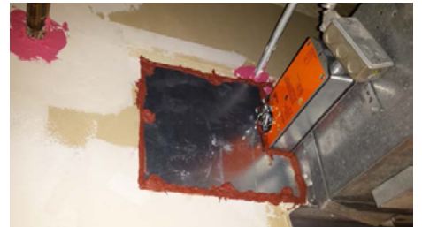
Figure 12.20 Detail of drywall repair.
