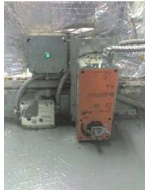
Figure 3.50: New Belimo FSNF120
