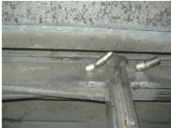
Figure 12.36 Rope connected damper
