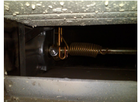
Figure 6.5: Detail of spring, arm, and fusible link
