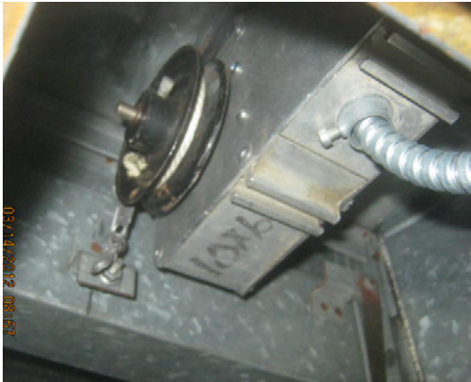
Figure 12.35 Guillotine damper
