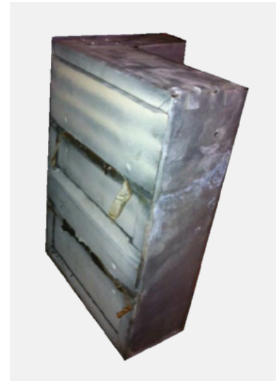
Figure 9.28: Prefco damper viewed from front
