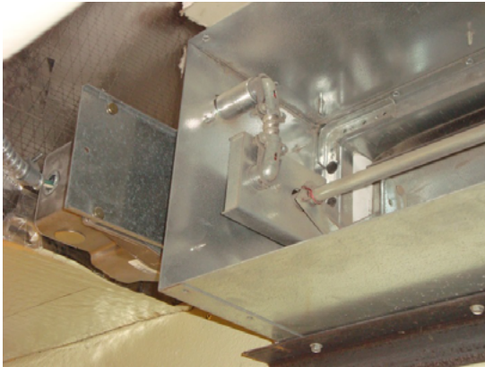
Figure 5.24: Typical damper and motor with auxiliary switch package
